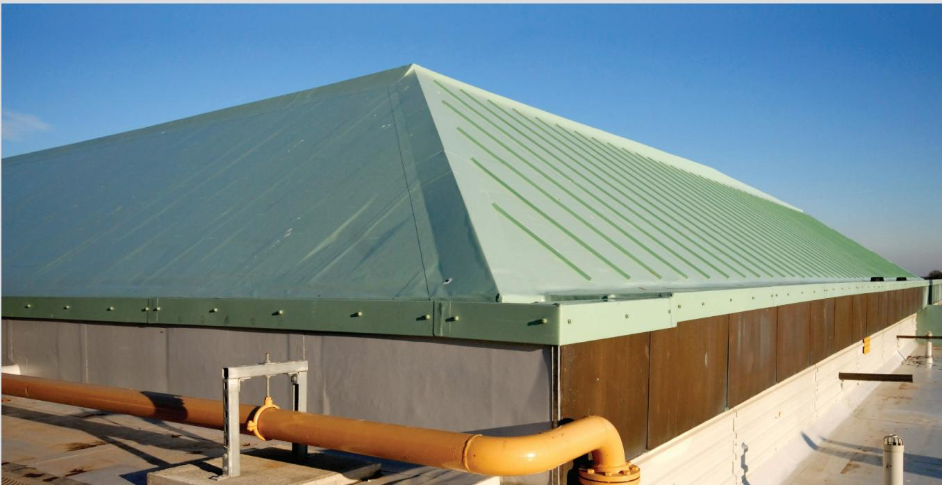
Roofing Contractors Cambridge Limited (RCC) carried out the refurbishment. Phase one saw the installation of Sarnafil's cold-adhered Light Grey G410-15EL membrane on the flat gym roof and other flat areas. In phase two, a year later, the swimming pool roof was refurbished in green Copper Patina membrane with a Decor Profile to replicate the traditional standing seam roof look in-keeping with the building's aesthetics.
